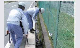
Local clean-up operation
