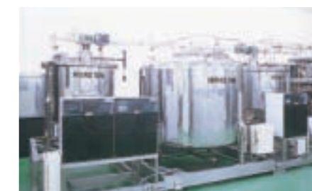
Developer Dilution Supply Equipment
