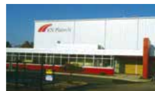
Receiving Numerous Orders of Deck Boards from Auto Manufacturers in the U.S.
