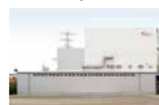
Okayama Functional Saccharide Plant, T Building
