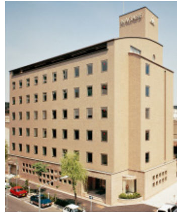
Nagoya Branch Office
