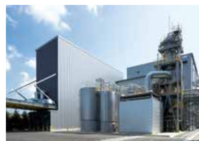
Okayama Functional Saccharide Plant, T Building
