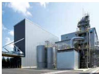
Okayama Functional Saccharide Plant, T Building (TREHA™ production)
