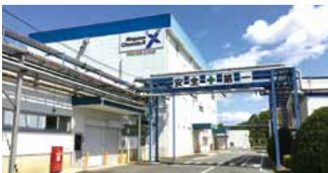
Nagase Chemtex Fukuchiyama Plant
