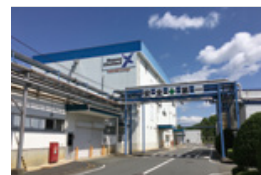
Nagase ChemteX's Fukuchiyama Plant
