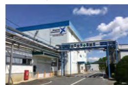
Nagase ChemteX's Fukuchiyama Plant
