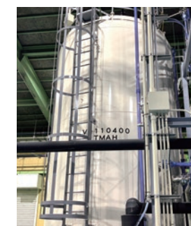
Semiconductor developer fluid (tetramethyl ammonium hydroxide) storage tank
